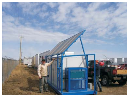
RAISING SOLAR PANELS
